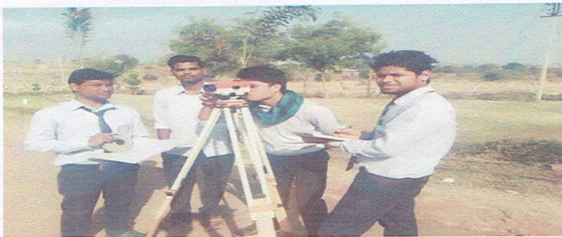
Image 2: Taking a reading on Bench Mark
