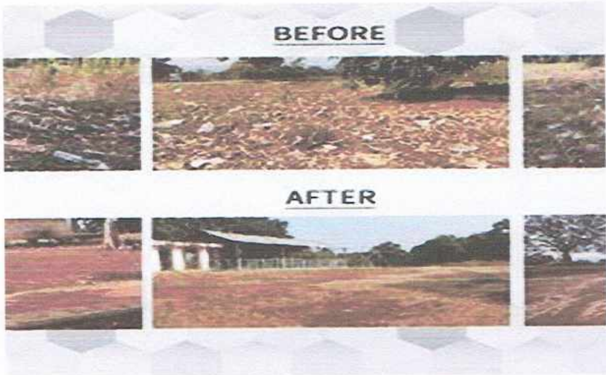
Photo 05:- Before and After Cleaning of Matoshri Vrddhashram Nilona by Student and Staff of Jagdambha College of Engineering And Technology Yavatmal.
