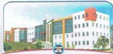
Jagadamba College of Engineering & Technology Arni Road, Yavatmal - 445001 (M.S.) INDIA
