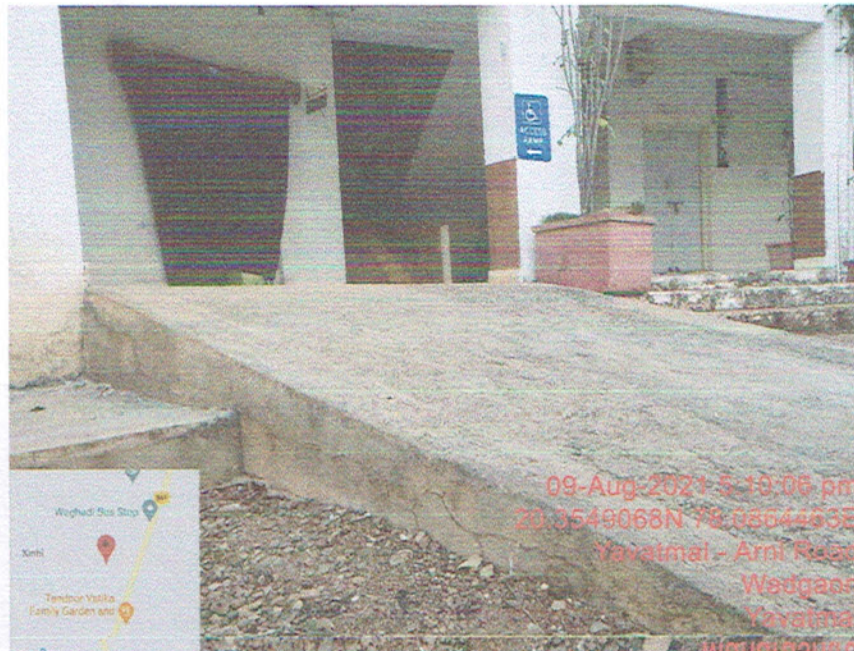
Ramp with Signpost
